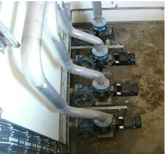
Pumpenleistung 90l/s = 5300l/min = 320m 3 /h
